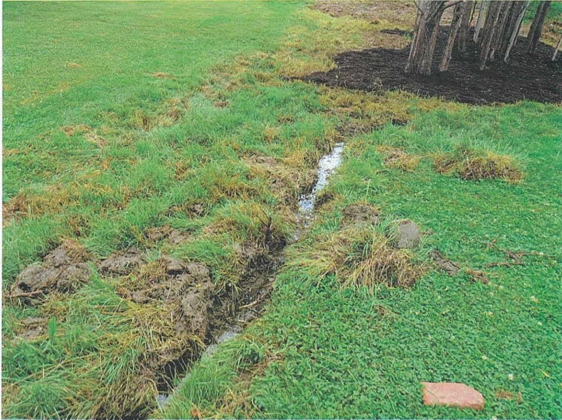
This picture was taken in July 2019 after one of CRC's many attempts to dry the wetland. You can see that there is flowing water in the hand dug trench. Note that the lawn has not been mowed because it is too wet for a mower. Note also the fresh bark mulch that CRC spread under the trees in an effort to soak up water.
