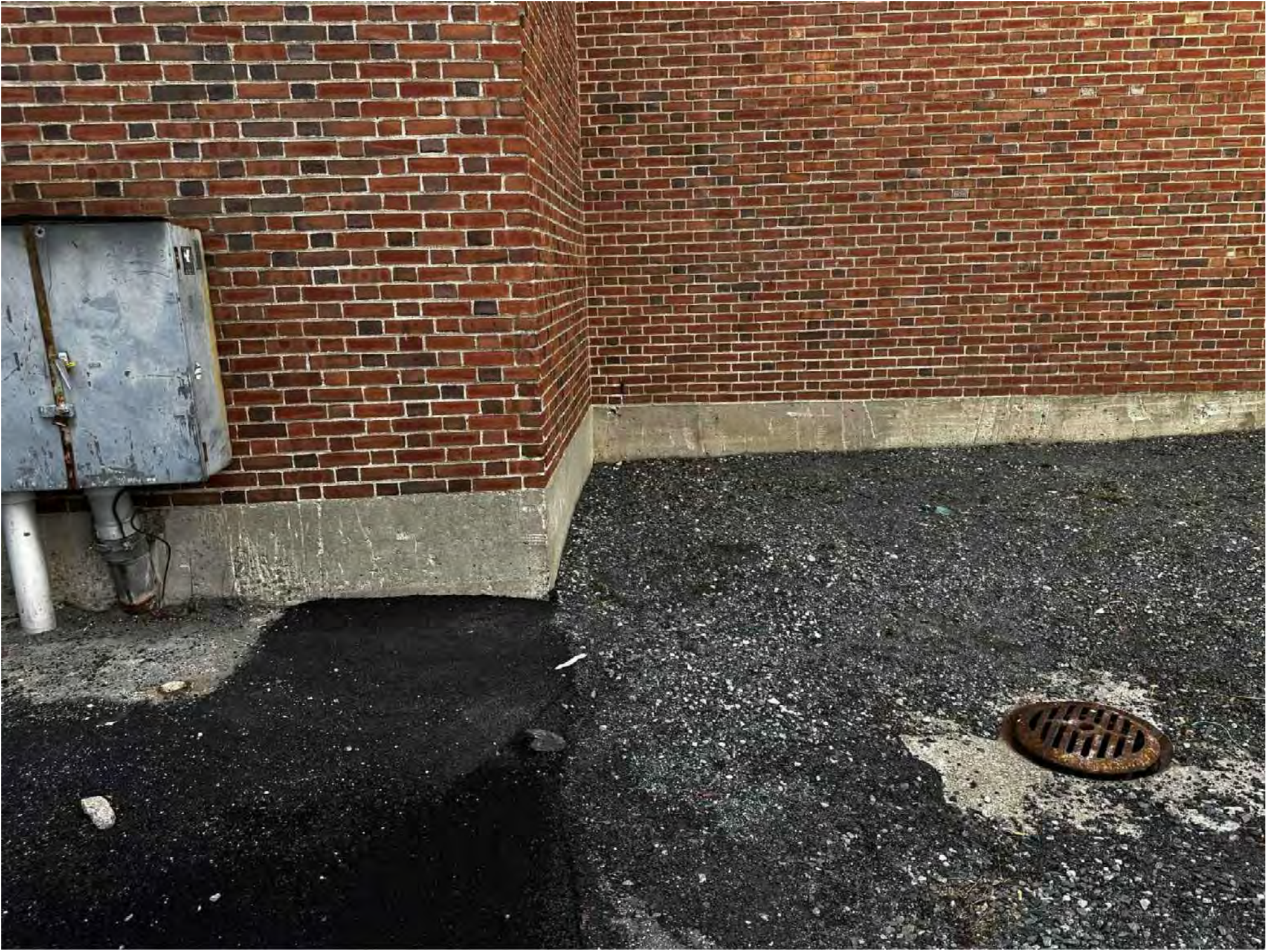
EXISTING CATCH BASIN TO BE INSPECTED AND GRATE REPLACED WITH NEW (DMH) DRAINAGE MAN HOLE COVER OR REPLACE ENTIRELY WITH A NEW DMH, SEE SHEET L1.1
