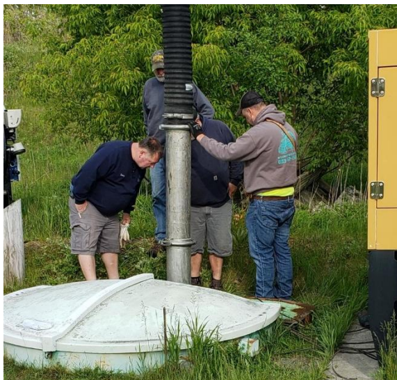
Pump Station #4 Wet-well cleaning
