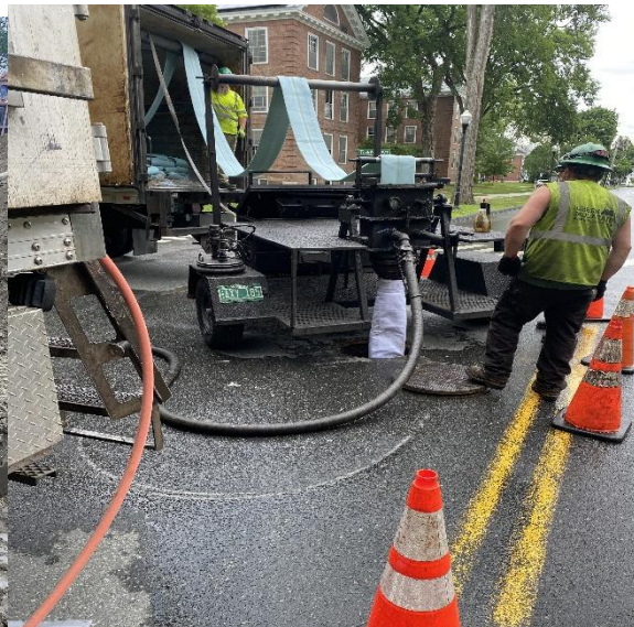
Slip-lining North Main Street Sewer
