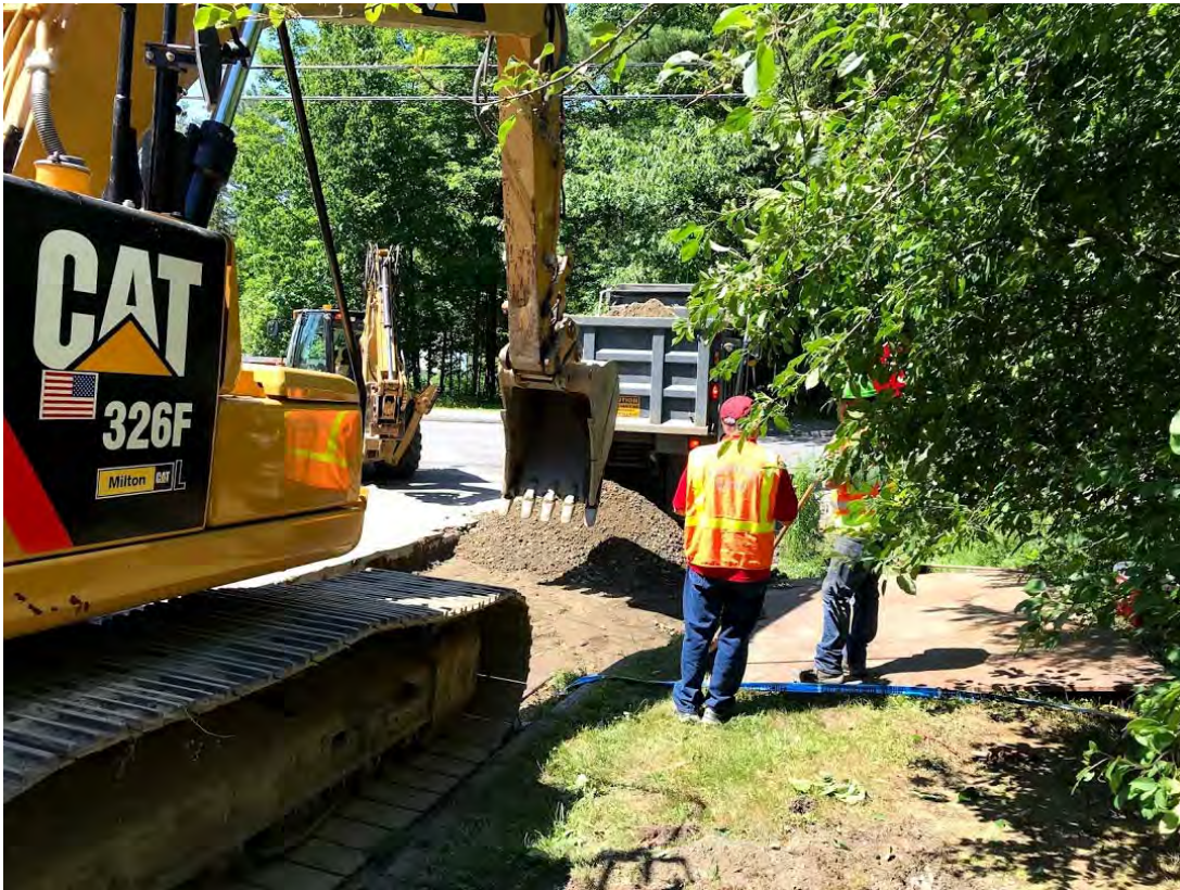
Water Main Replacement on Low Road
