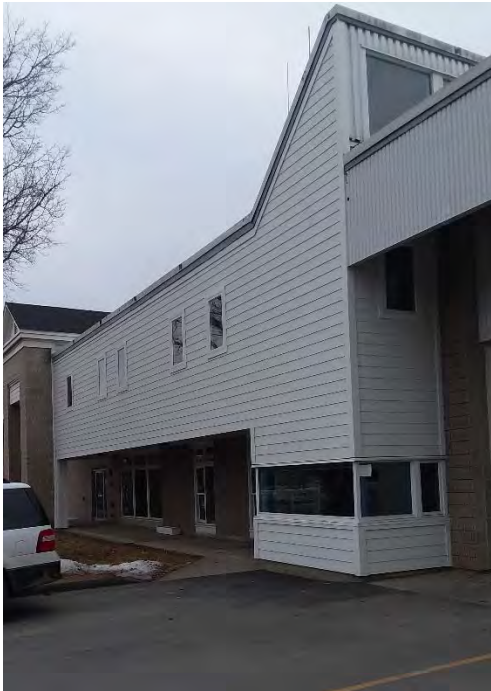
New PVC Siding and Energy-Efficient Windows at Public Safety Building
