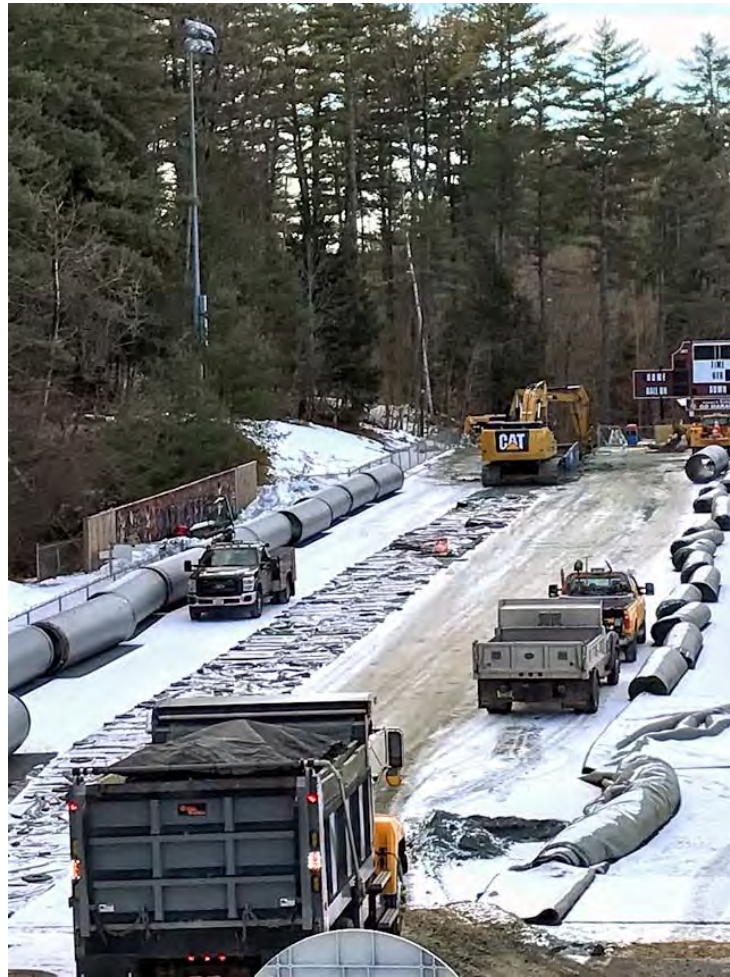
Hanover High School Drainage Work
