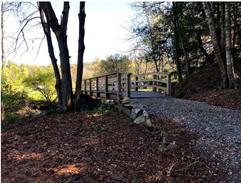
Farr Field Bridge
