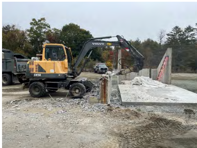
Photo showing the removal of a structure and the construction of the housing for the new grizzly
