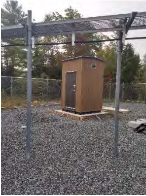
Canaan Radio Building
