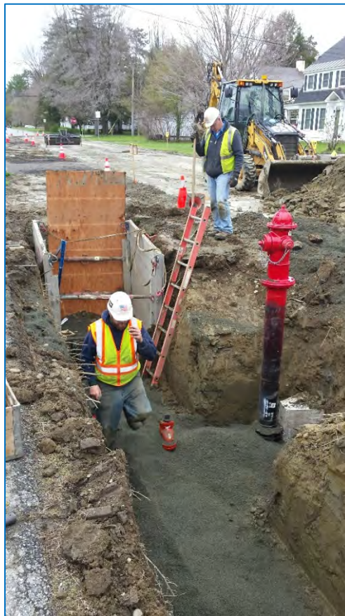
Water Main Replacement on South Balch Street
