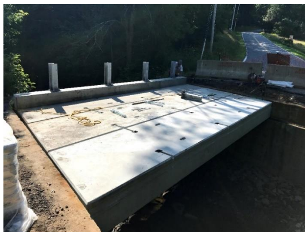
Stevens Road Bridge
