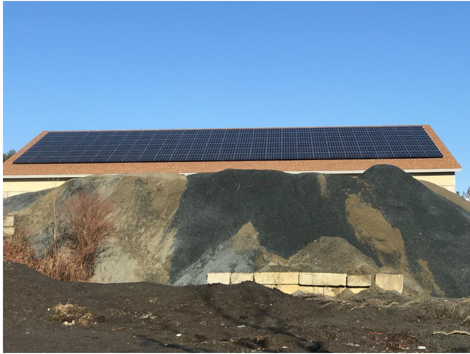
Solar on Winter Materials Barn @ Public Works
