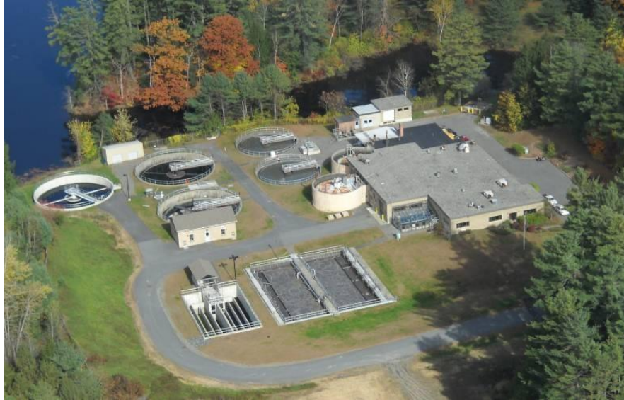
Facility aerial view
