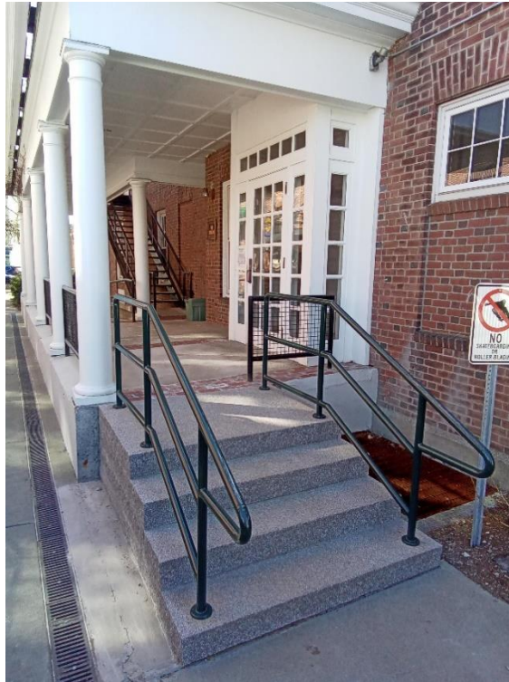
Town Hall Stair Replacement
