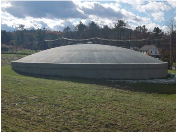
Grasse Road 1.0 Million Gallon Storage Tank
