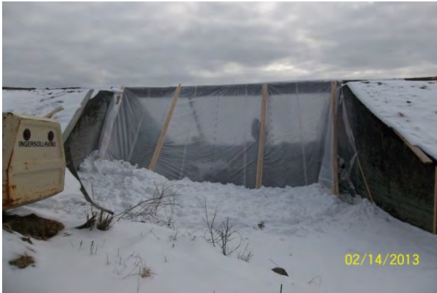
Parker Reservoir Spillway Winter Construction
