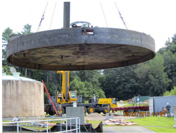
Old Digester Cover Removal
