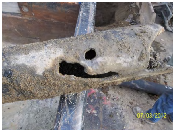
1893 Pipe from Lebanon Street
