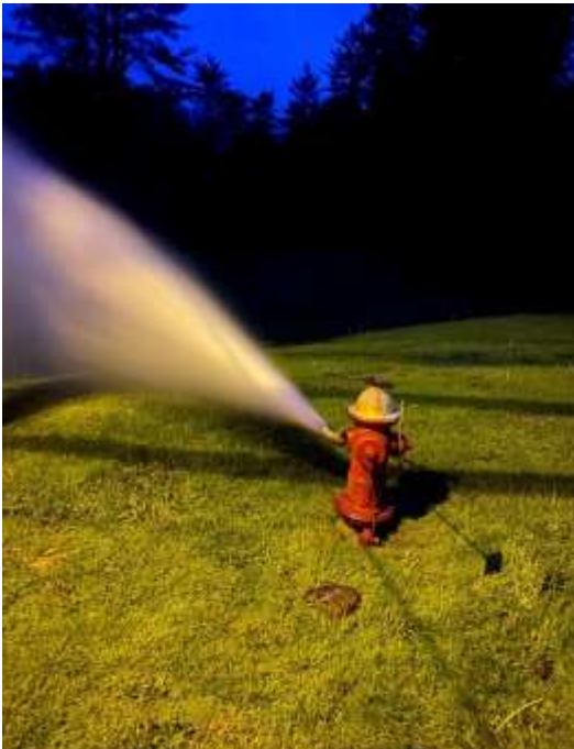
Hydrant Flushing
