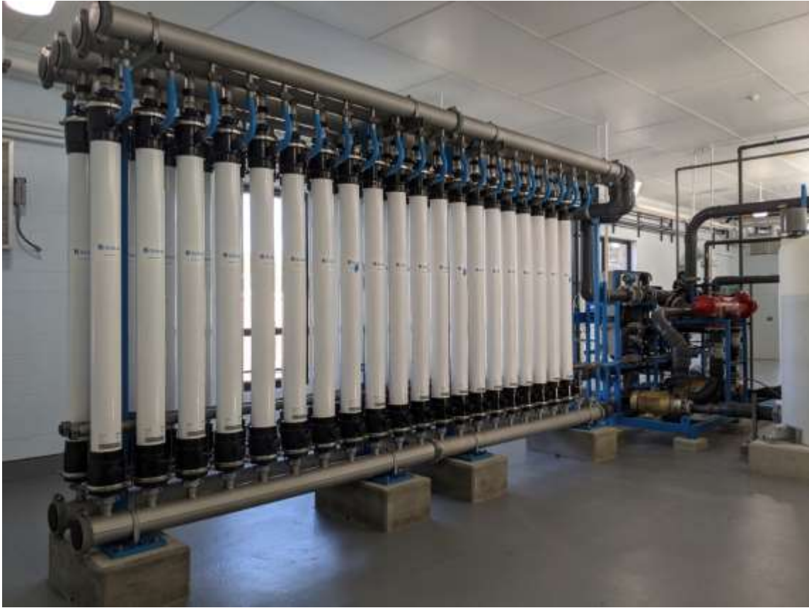
Filtration module replacement at Water Treatment Facility
