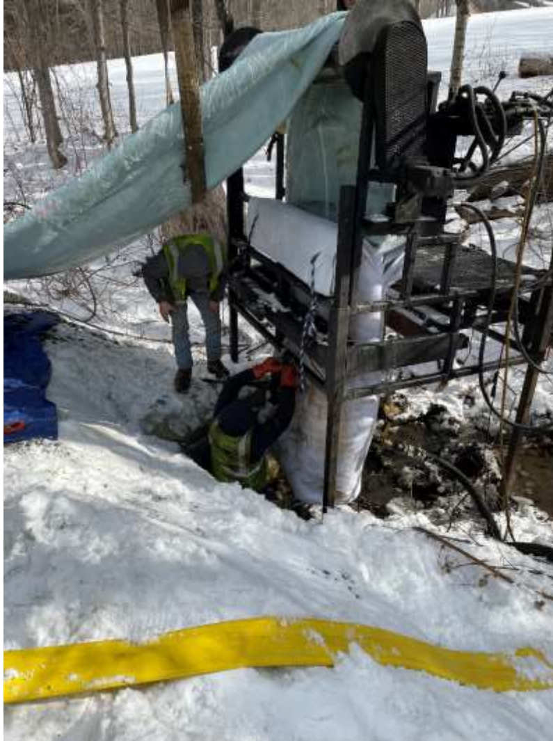
Culvert Sliplining on Stevens Road
