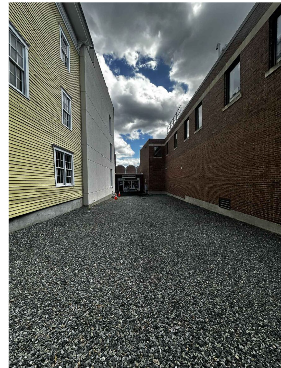
VIEW FROM MAIN STREET ENTRANCE GRAVEL TO BE REMOVED, SEE SHEET L1.1
