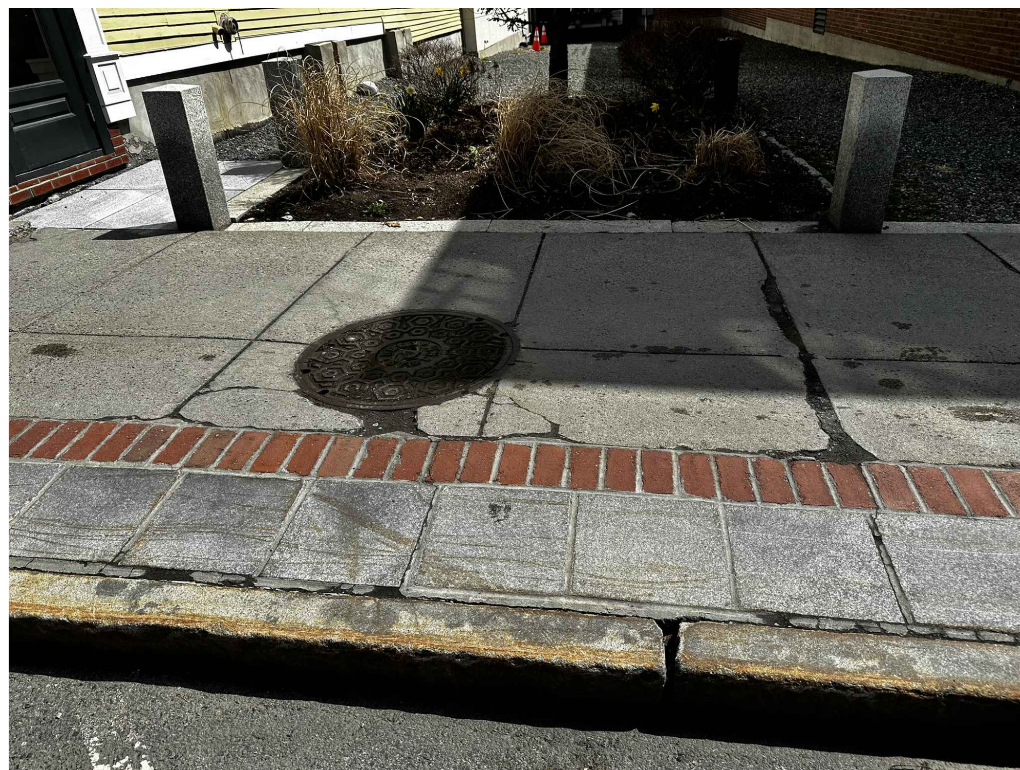
VIEW FROM MAIN STREET 4"X8" AND 12"X12" PAVERS TO REMAIN. VERTICAL CURB, CONCRETE, MULCH BED, ALL PLANTINGS, AND ALL GRANITE POSTS AND PAVERS TO BE REMOVED. SEWER MAN HOLE TO BE RESET AT EXISTING GRADE. SEE SHEET L1.1
